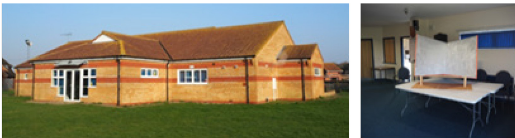
Figure 10: Brick building imaged with calibration target inside.
